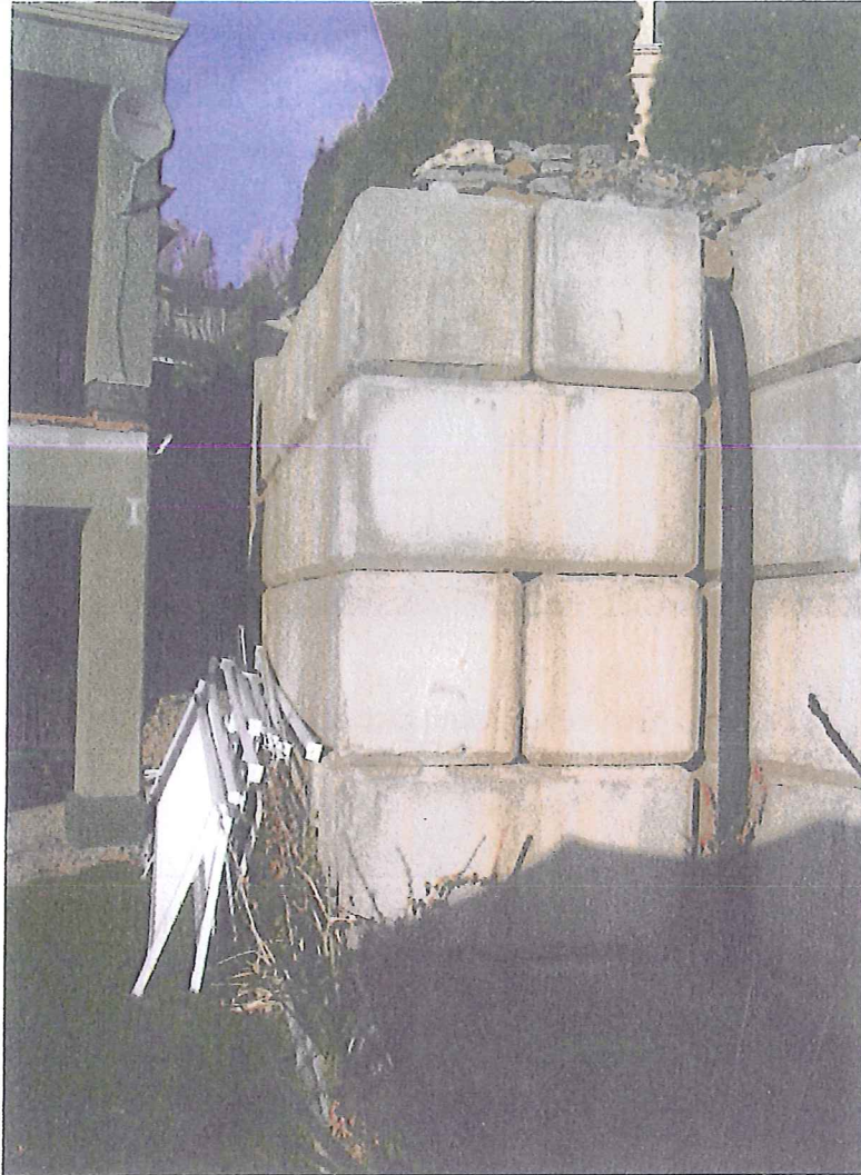
Photo 2: Downslope corner of the wall. There are no visible deformations in this wall segment.
