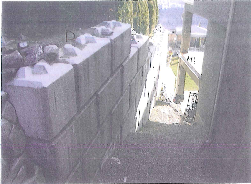
Photo 1: View of the south face of the retaining wall.
